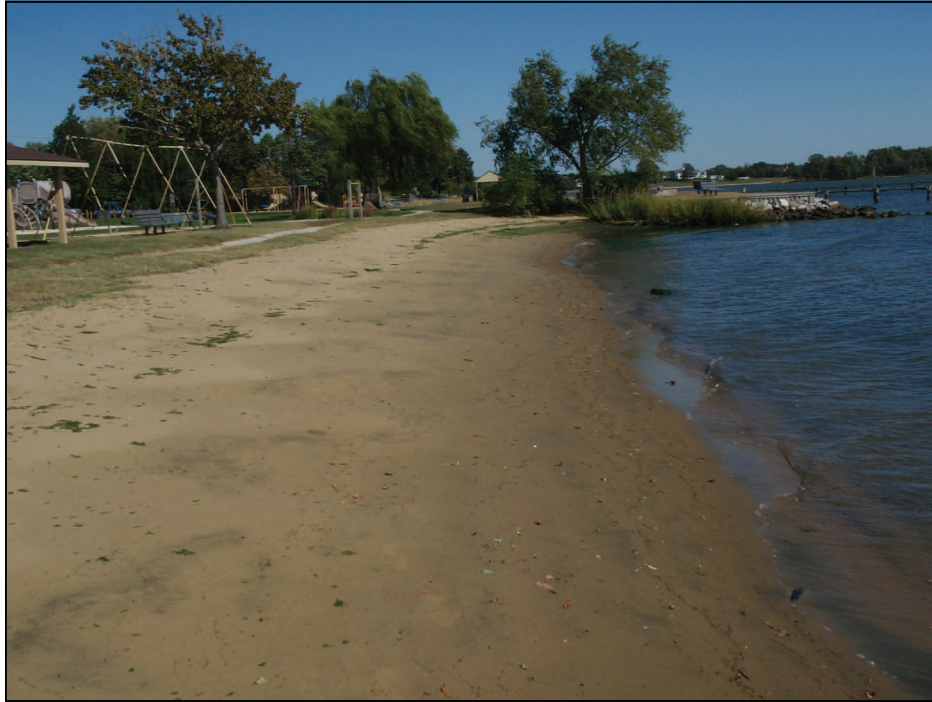
Figure 17. Gradually sloping natural beach area looking northeast toward bulkhead. This bulkhead inhibits longshore transport and results in shoreline accretion/up-drift deposition.
