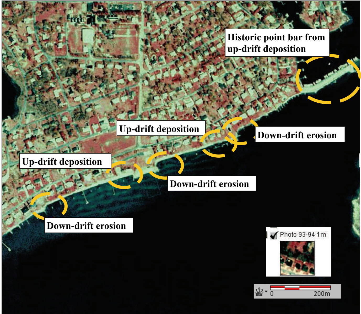
Figure 12. Material is transported along Hillsmere Shoreline into Duvall Creek. Current bulkheads inhibit this transport leading to deposition along the southwest bulkhead. Classic up-drift deposition and down-drift erosion normally associated with structures that interfere with littoral transport seems to be occurring at Hillsmere.
